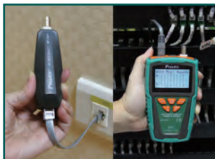
Verify LAN/ Telephone / Coaxial cable condition
