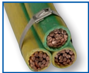
Stainless Steel Cable Tie Tensioned/Cut/No sharp edges
