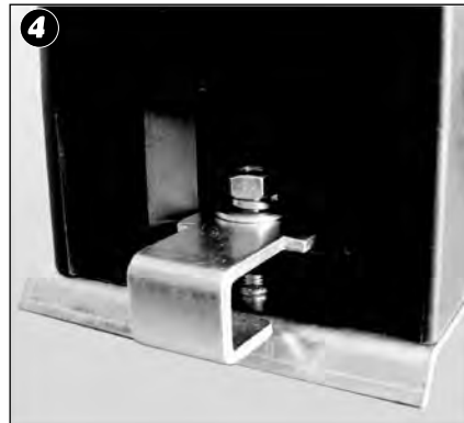
4 Re-fasten the washer and nut to the retaining stud to secure the bracket.
